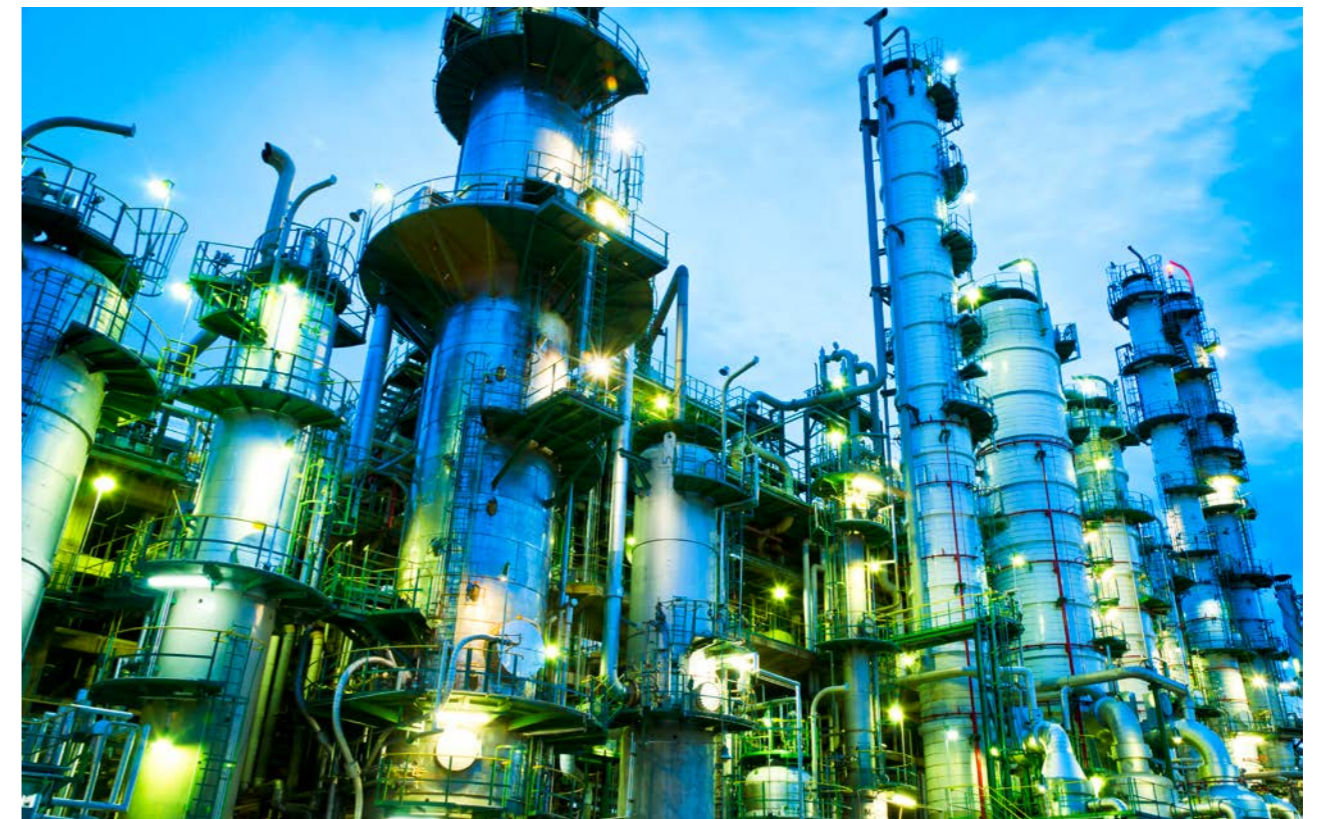
↓ A great deal of know-how and well-trained specialists could be found and still can be in the Central German chemical triangle around Halle/Saale, Merseburg, and Bitterfeld. The locations remained, and investments were made for their modernization. Photo: mmmx / AdobeStock
