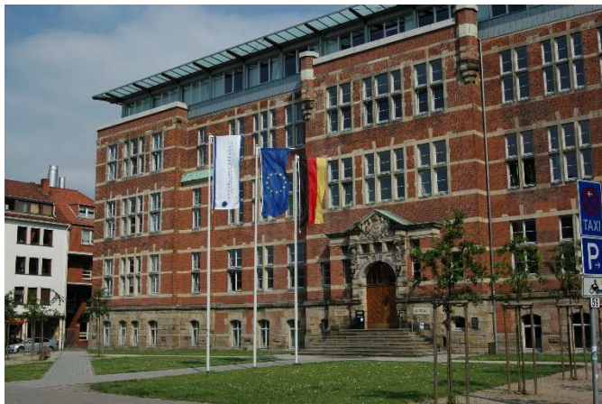
Neustadtswall: M Building
